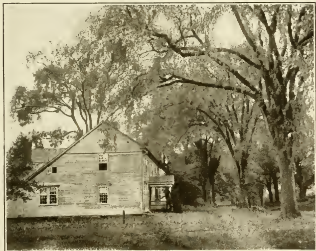
FRARY HOUSE, DEERFIELD
